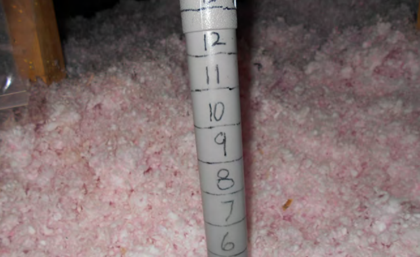
(left) HERS rater John Richau found less-than-best practice attic insulation. The insulation installers had to return to bring the level up to the 13-inch standard. (right) Upon inspection of shower-tub units HERS rater John Richau determined that 14 were installed improperly, without water-resistant backer board. All 14 had to be removed and re-installed properly.
